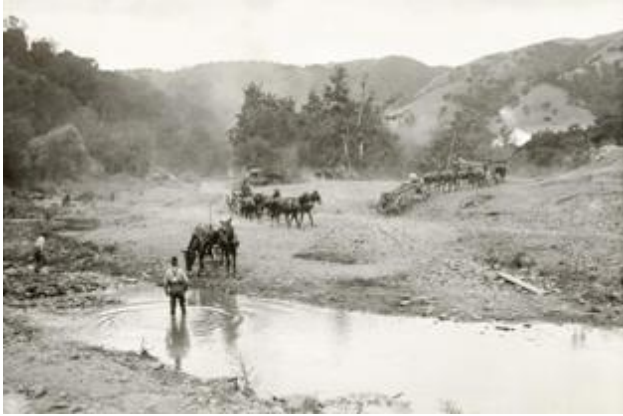
Workers conducting initial excavation work on the Calaveras Dam in the early 1900s.
